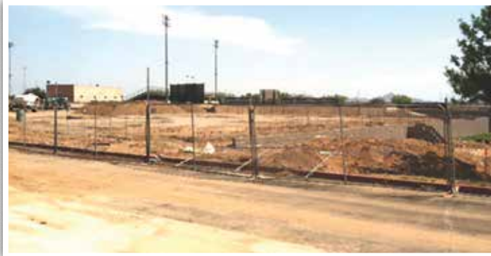
Pinnacle High School under construction
