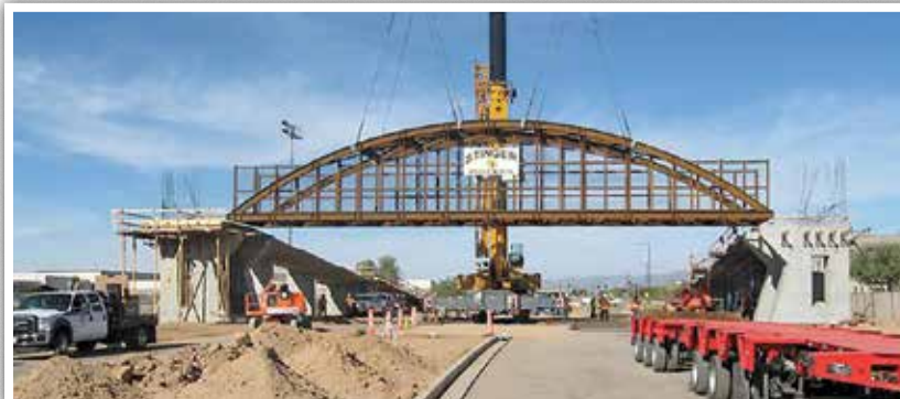
Black Mountain Boulevard/SR 51/Loop Extension under construction circa 2015
