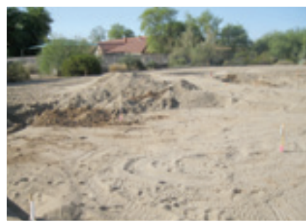
Future ramada location and reconditioned volleyball courts
