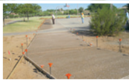
New concrete sidewalk connection
