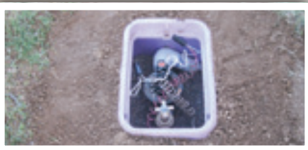
New irrigation valves upgraded in park.
